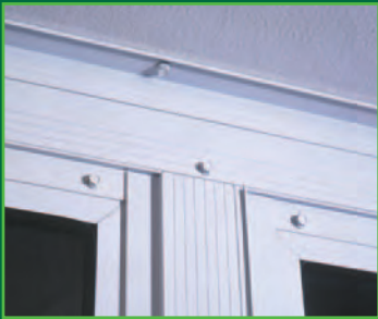
EXPOSED FASTENERS Unfinished appearance.
