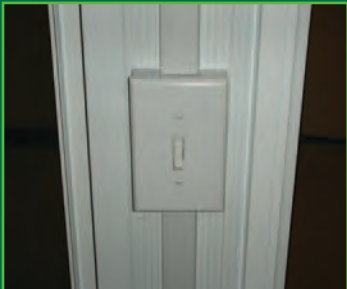
SURFACE MOUNT Unsightly conduit for electric, cable, telephone and sound system lines.
